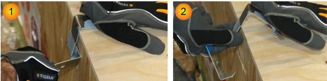
Fig. 5: Removing the metal brackets using the lever. Start by sliding the lever under one of the metal bracket's grooves and lift it away from the wooden wall while holding the top of the bracket (1). Remove the bracket as shown in (2)
